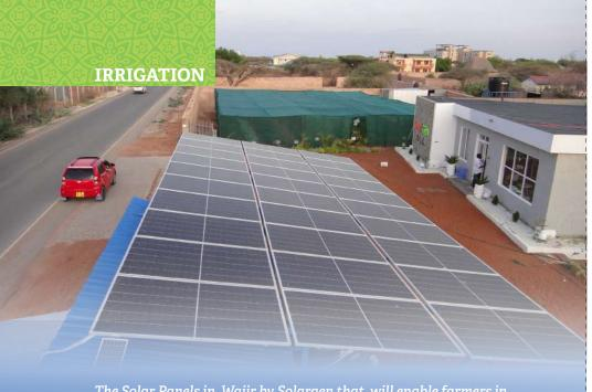
The Solar Panels in Wajir by Solargen that will enable farmers in the region harness solar energy to power their water pumps instead of using costly dieselpowered generators while the drip irrigation will ensure optimal use of water. Photo Credit: Solargen.
